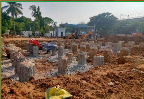
Pile cap works under progress in Chennai centre.
