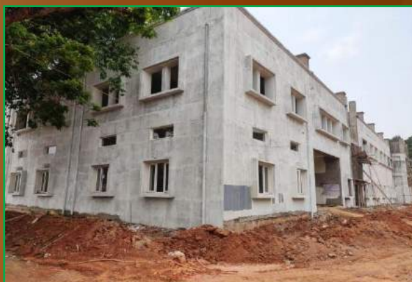
Construction of academic cum workshop building Ranchi centre.
