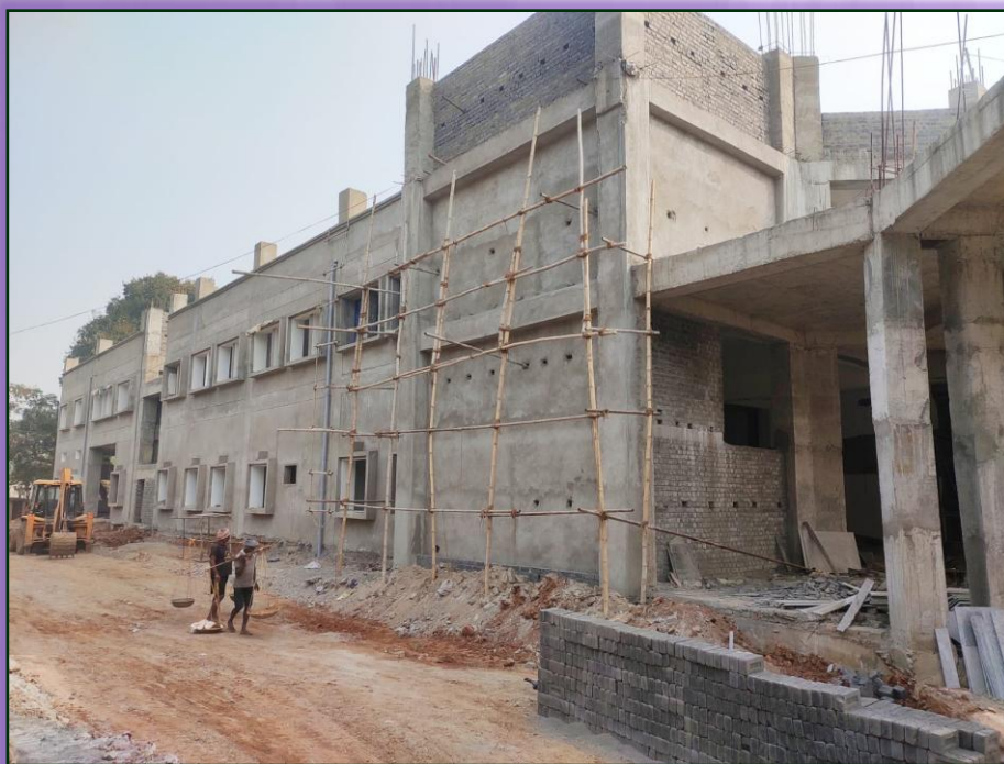
Construction of Academic Cum Workshop Building at Ranchi centre
