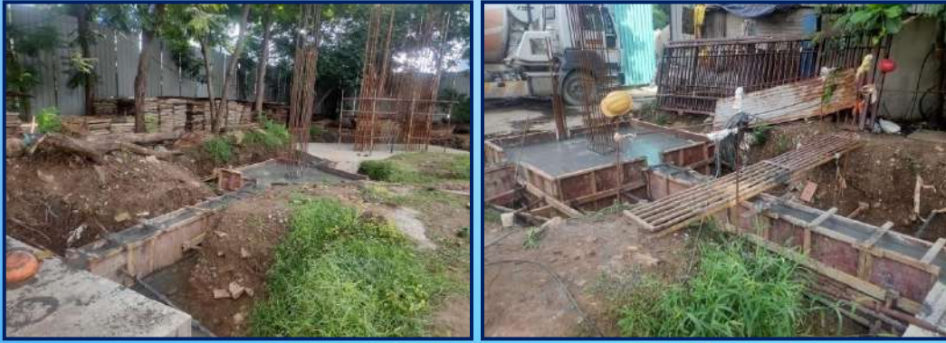
New Technology Centre - Pile cap casting work at Chennai centre.
